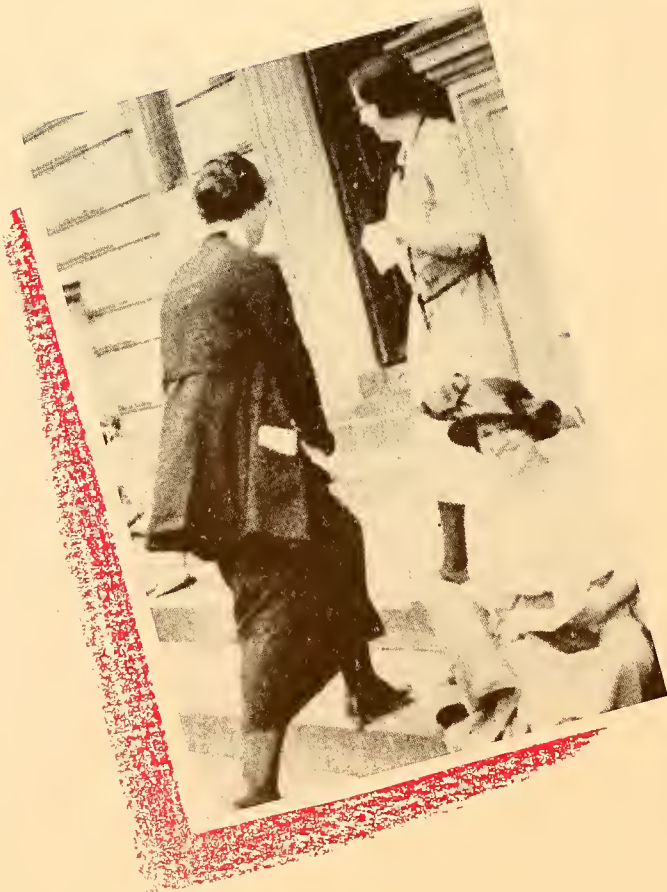
The front of the building was still the same when students and faculty walked in to class in the morning many years ago.
